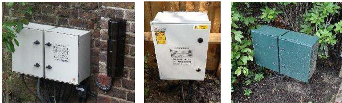
*Enclosures should be securely installed, above ground, in a location that is accessible and serviceable to the system as well as out of harm's way. They should be lockable and all connections undertaken so that the integrity of the enclosure is withheld (all access points vertical from the underside, so that water ingress is least likely).*
